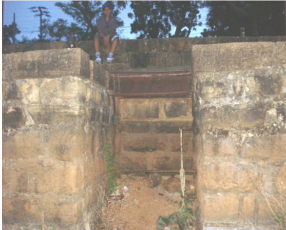
Figure 5 Present Remains of the High-Level Sluice Inlet (Bisokotuwa) of the Minneriya Tank, Locally Known as the Miggolla Sluice (Photo September 2009).
