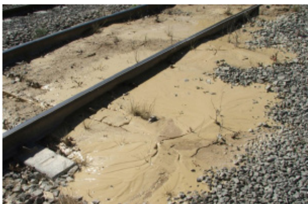
Photo 4: Ballast particles are clogged due to mud pumping
