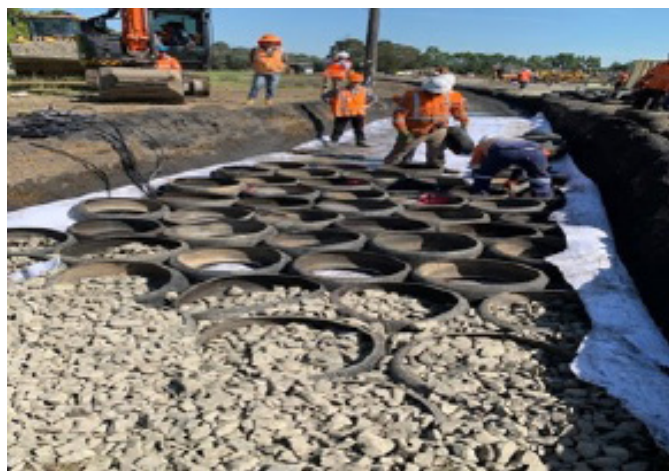
Photo 3: World's First Rubber Tyre Cell Foundation for Railways at Chullora
