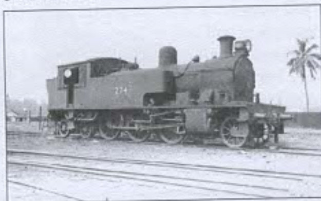
• Figure 6: Class D2 2-6-4T Tank Steam Locomotive.
