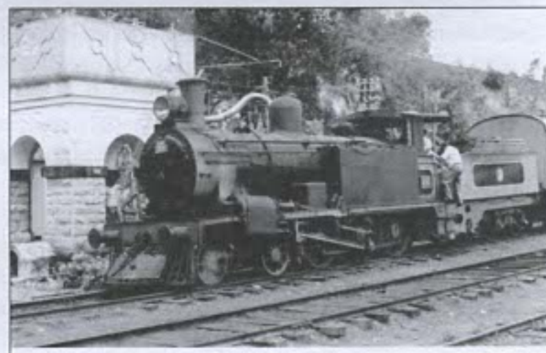
• Figure 2: Class B2 4-6-0 Tank-Tender Steam Locomotive.
