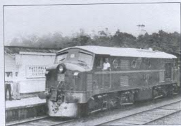
• Figure 8: Class M1 A1A-A1A 1,000 hp Brush-Bagnall Diesel Electric Locomotive.
