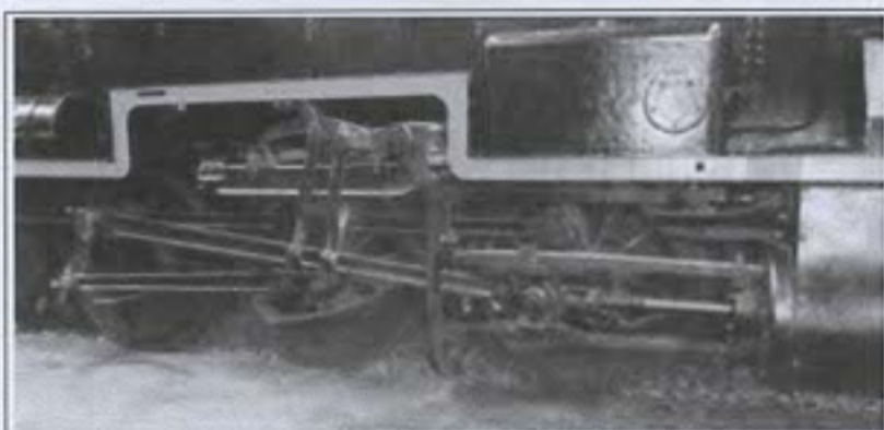
• (Figure 4) Southern Valve Gear.
