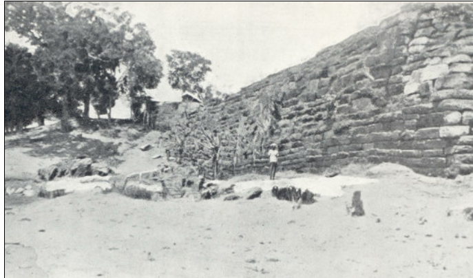
A section of the ancient spill, Kala-wewa tank looking upstream. This stupendous work of hammered granite, excellently dressed and at the top mortised, existed in a contracted form for centuries before it was enlarged in A.D. 477.
